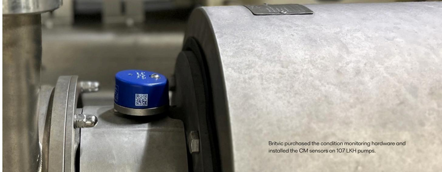
Britvic purchased the condition monitoring hardware and installed the CM sensors on 107 LKH pumps.
