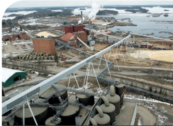
The Kaukas facilities, close to the Russian border, produce 590,000 tons of LWC (lightweight coated) paper annually and 720,000 tons of bleached sulphate pulp.
