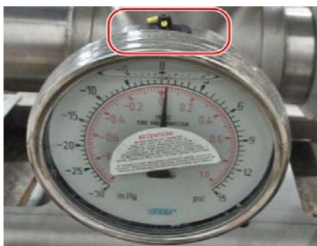
Gauge seal valve on top of gauges
