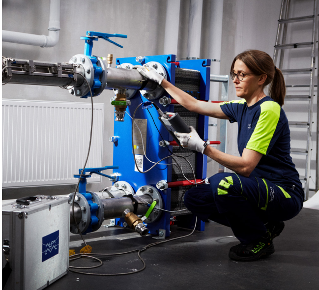
Performance assessment being performed on a plate heat exchanger. Example photo of performance assessment service.
