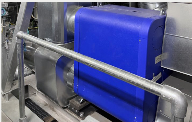
Condenser and subcooler - CBH410
