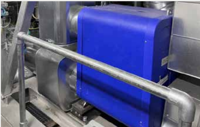
Condenser and subcooler - CBH410
