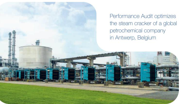
Nine Alfa Laval M30 units are responsible for cooling down the process water of the steam cracker.
