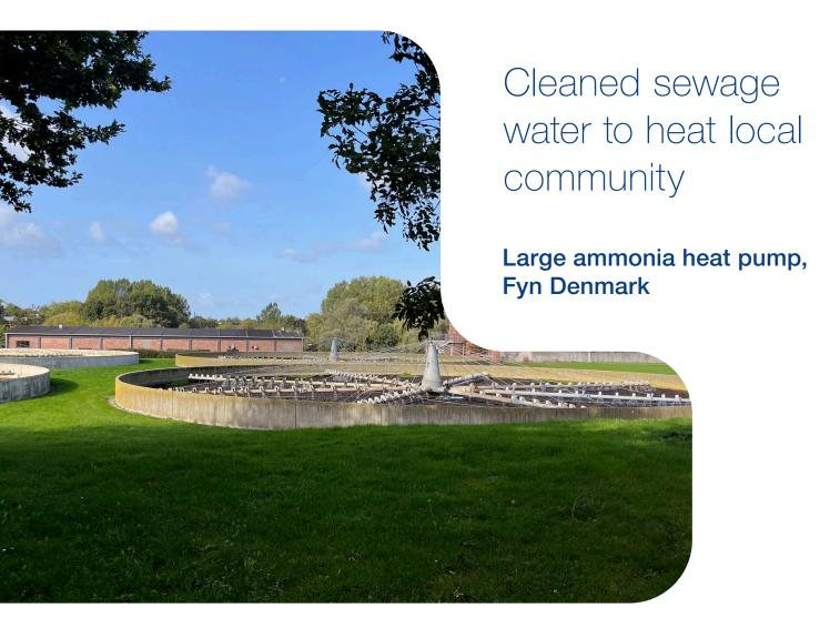
The installation of heat pumps at wastewater treatment plants has a huge, but rarely exploited, potential. The heat pumps can utilize the wastewater's energy that would otherwise have been wasted and thus send greener and cheaper energy into the district heating system.
