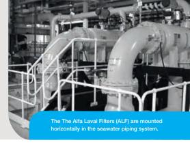
The Heysham plant's seawater filtration system uses water from Morecambe Bay. However, the bay is relatively shallow and sandy, which means the filtration system has to remove sand as well as marine life and shell debris.
